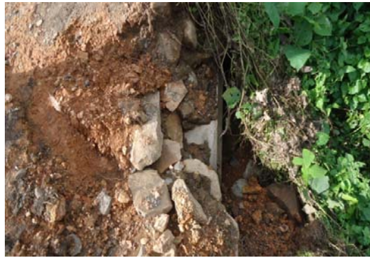
Fig.5.8.11:Pipe culvert at 406+400 (Choked)
