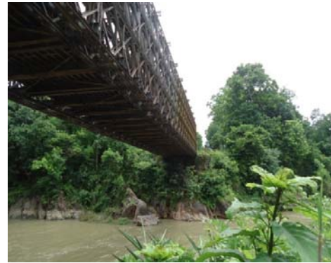
Fig.5.8.12:Bridge Bailey Type Super structure at Indo Myanmar Border
