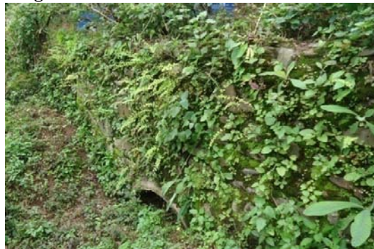
Fig.5.8.9:Pipe culvert at 393+040 (Partially chocked)
