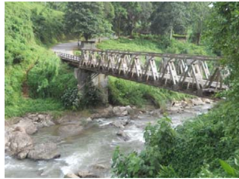
Fig. 5.8.4: Minor Bridge With Bailey type superstructure at 407+700
